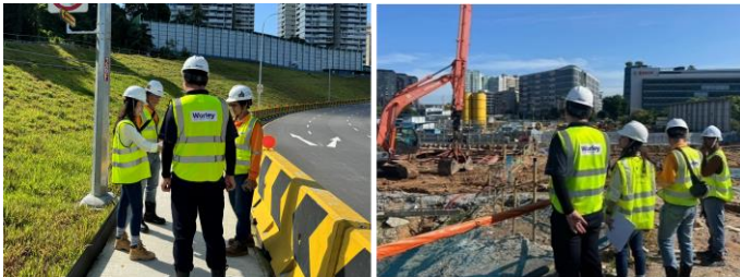
Figure 28 The author with Qualified Person Supervision (GEO), Resident Engineers, Instrumentation Contractor on site-walk
