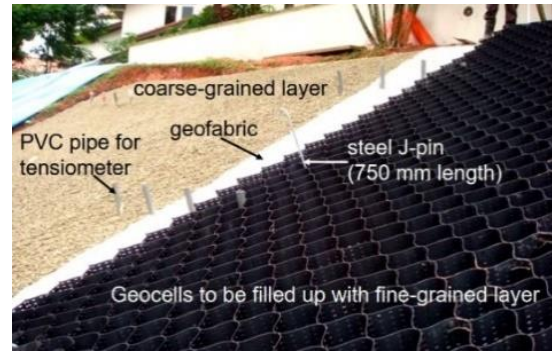
Figure 26 Geocell arrangement (Satyanaga et al, 2019)
