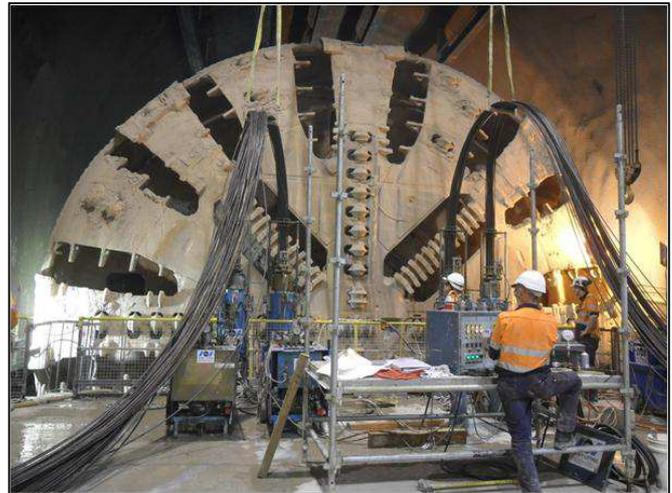
**Figure 7 - Lowering the TBM Shield**
