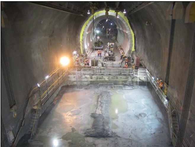
**Figure 8 - Final burial with the top of the TBM Shield visible**
