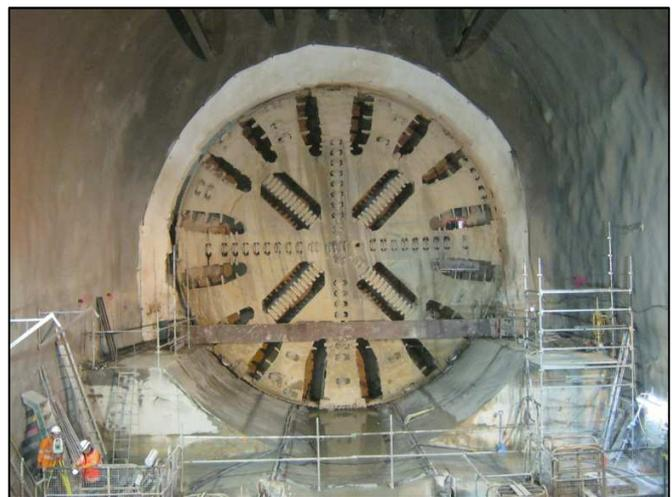
**Figure 5 - Restraint Beam was installed shortly after breakthrough**
