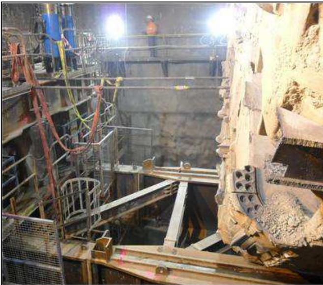
**Figure 6 - Pulling the TBM Shield forward on the Steelwork**
