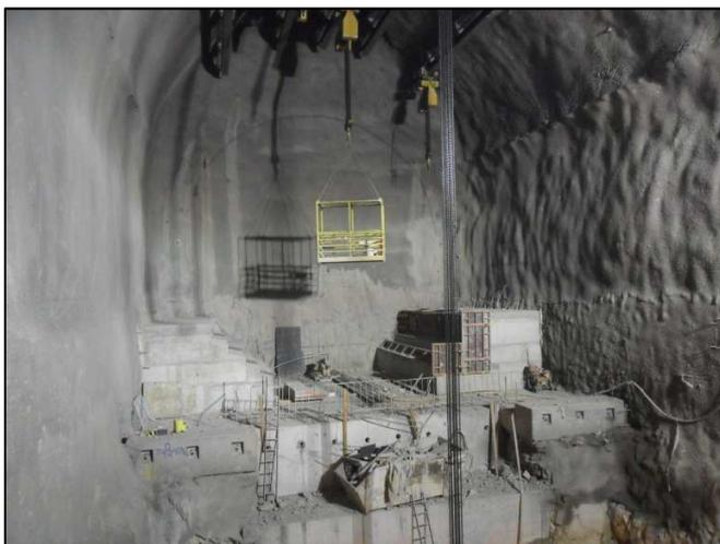
**Figure 3 – Construction of Burial Pit showing Rear Edge Beam and the Concrete Cradle Billet**
