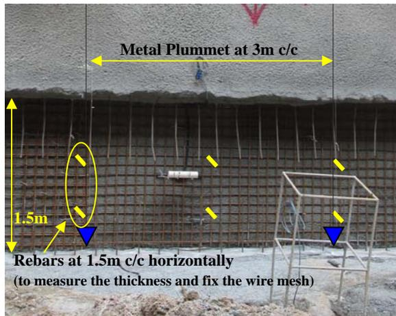
Figure 8. Measuring system of shotcrete profile
