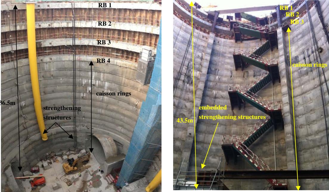
Figure 7. Completed sprayed shotcrete structure of S-Shaft and cast in-situ concrete structure of PIE Shaft
