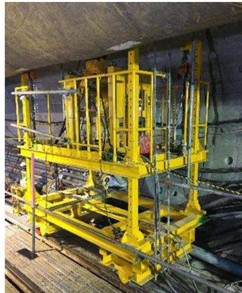
Figure 17 T207 Raito Working Platform
