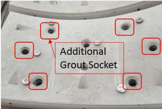
Figure 14: T207 Additional grout ports arrangement
