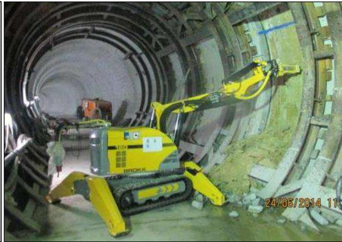
Figure 12: C927 Excavation of CP using remote controlled excavator
