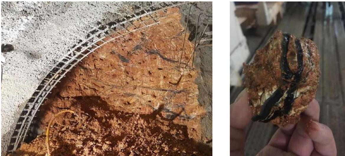
Figure 19: Adit Tunnel excavated face and soil sample showing grouting veins
