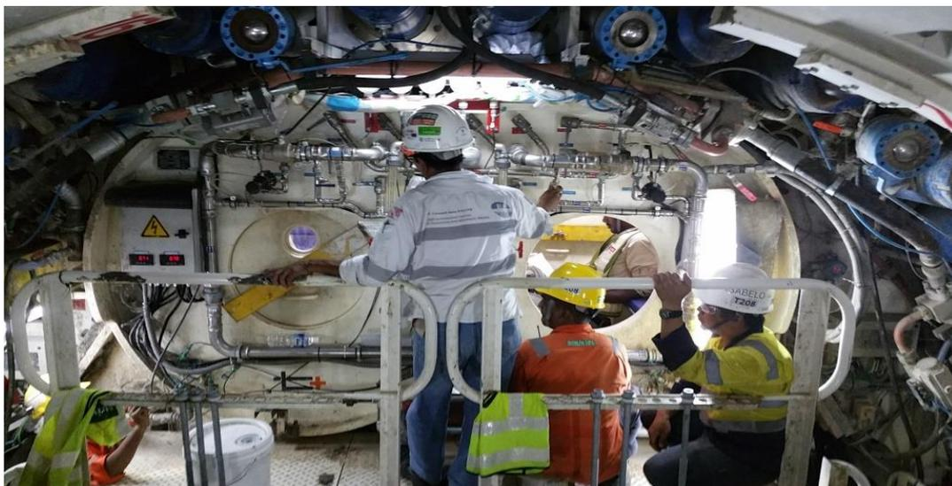
Figure 2: Dual manlocks provided direct access into the working chamber for CAWs. Prior to the start of a CHI, both manlocks need to be pressure tested for any leakage as shown above.
